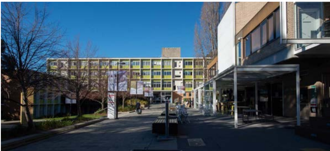
Figure 27: The area in front of the University Centre looking towards the former Arts Building.
