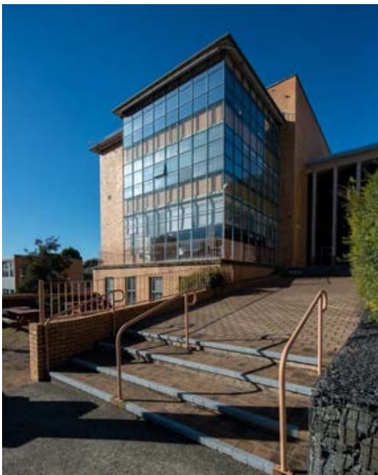
Figure 16: Chemistry Building main entry and glazed curtain wall northern façade.
