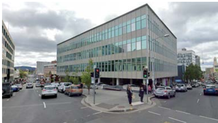
Figure 30: Google Streetview image of the library from the corner of Murray Street.
