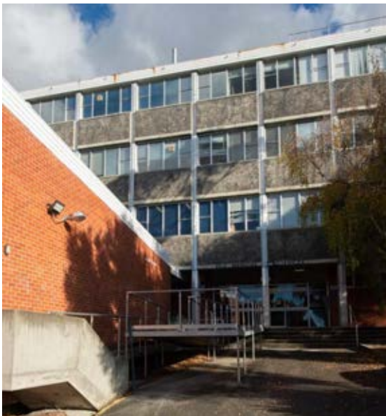
Figure 19: Medical Sciences Building with pre-cast spandrel panels and a later lecture theatre addition to the left.
