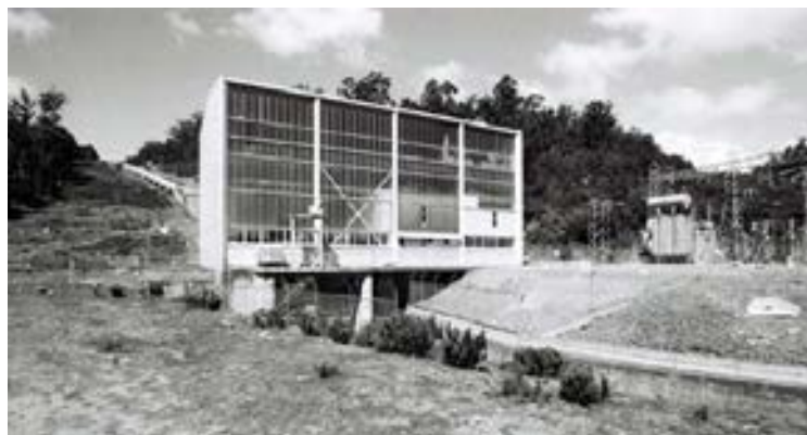
Figure 42: Lake Echo Power Station with its simple curtain wall form with brick solid end walls. Paul Davies.
