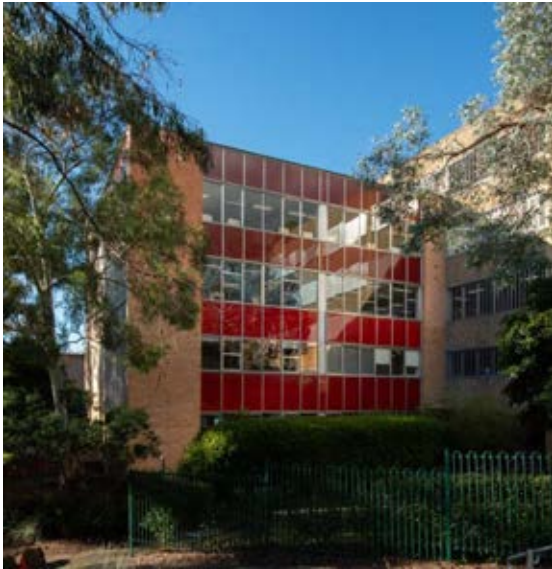
Figure 18: Morris Miller Library curtain wall façade set between brick end walls of the north-south wing.
