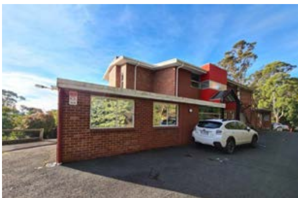
Building 38 – Research House South-western facade Source: Paul Davies Pty Ltd
