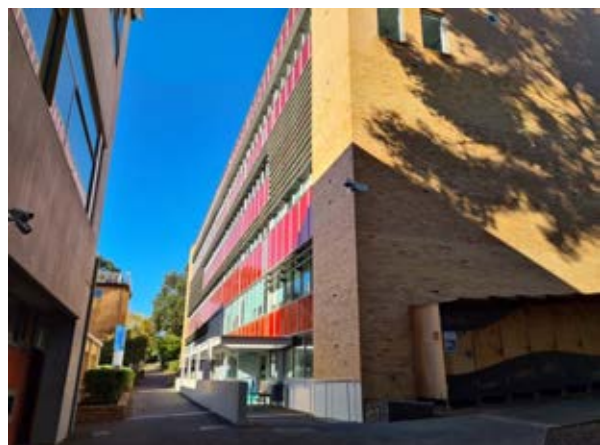
Building 23 – Library, Morris Miller North-western corner Source: Paul Davies Pty Ltd
