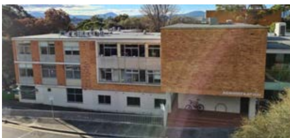
Building 22 – Administration Building Overview of the Administration Building from the hill to the south of Churchill Avenue Source: Paul Davies Pty Ltd
