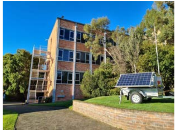
Building 14 - Mathematics Western façade Source: Paul Davies Pty Ltd
