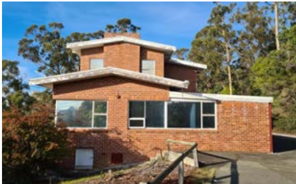
Building 38 – Research House North-western facade Source: Paul Davies Pty Ltd
