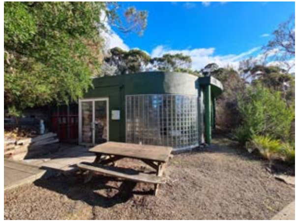
Building 36 – Herbarium, Tasmanian North-eastern corner Source: Paul Davies Pty Ltd
