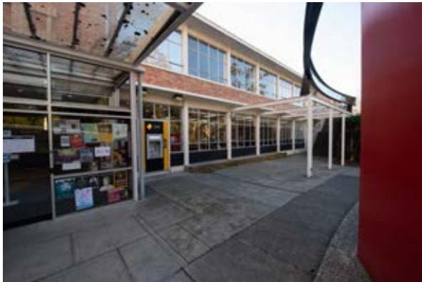
Building 21 – Tasmania University Union Eastern Façade – Main Entrance facing Dobson Road Source: Paul Davies Pty Ltd
