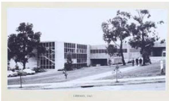
Building 23 – Library, Morris Miller
