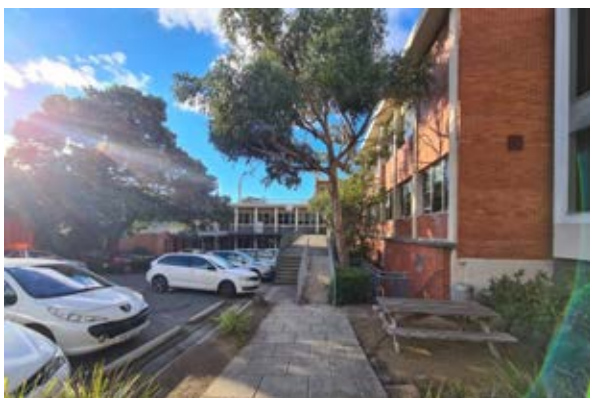
Building 34 – Life Sciences Building Southern and western facades Source: Paul Davies Pty Ltd
