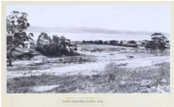
Building 21 – Tasmania University Union (Union Building) 1958 black and white print Under construction Source: University of Tasmania, Collection UT460 – Pictorial History of Sandy Bay Campus Buildings; Item 11
