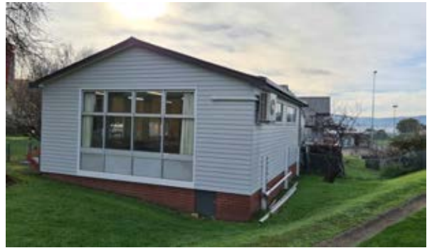
Building 53 – Childcare Cottage South elevation Source: Paul Davies Pty Ltd
