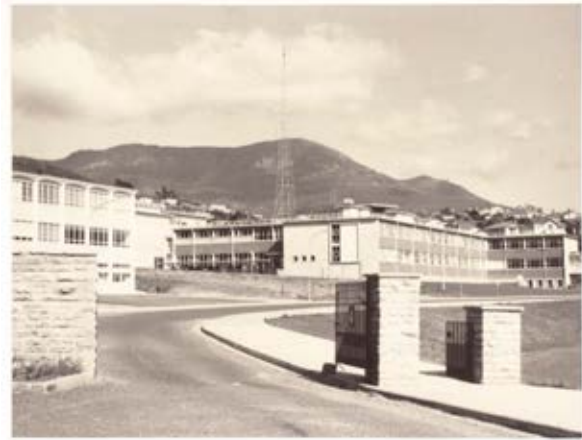
Building 8 – Engineering Building
