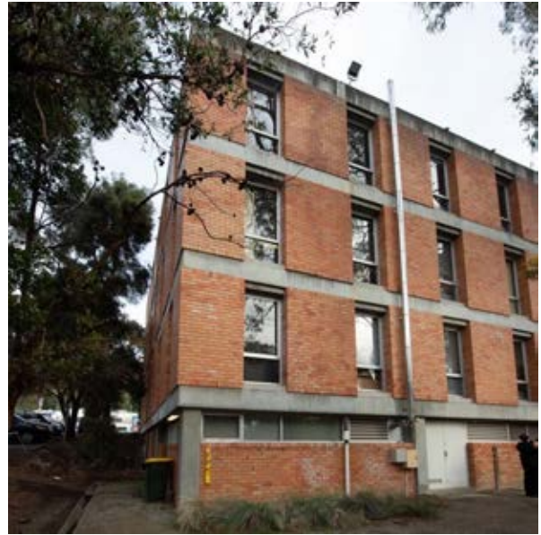
Building 29 – Humanities Building North-eastern corner Source: Paul Davies Pty Ltd
