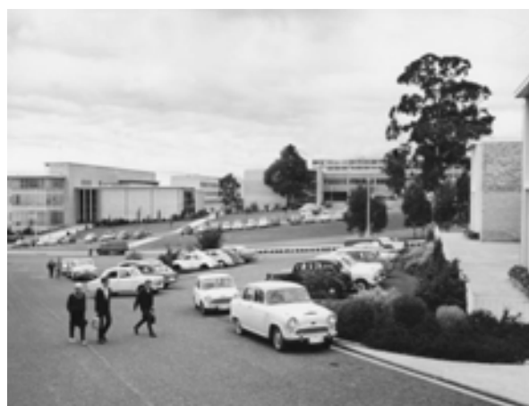
Building 23 – Library, Morris Miller
