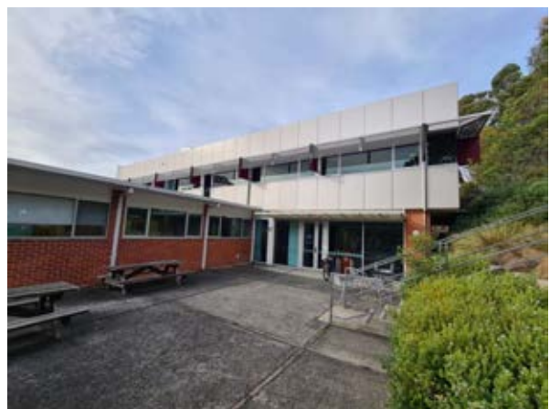
Building 32 – Corporate Services Building Western façade of the south-eastern wing Source: Paul Davies Pty Ltd
