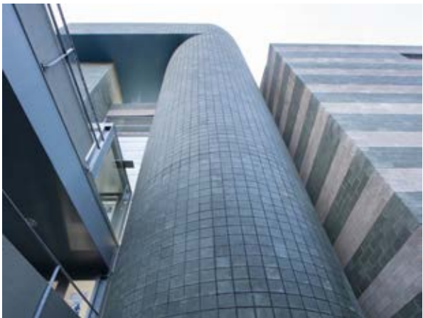
Building 10 – Centenary Building Column Detail Source: Paul Davies Pty Ltd
