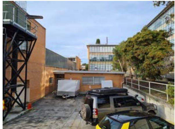
Building 11 – Engineering Workshop 1988 southern extension Source: Paul Davies Pty Ltd
