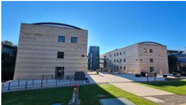
Building 10 – Centenary Building Southern facade Source: Paul Davies Pty Ltd
