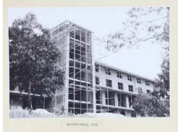
Building 40 – Hytten Hall 1958 black and white print Under Construction, northern facade
