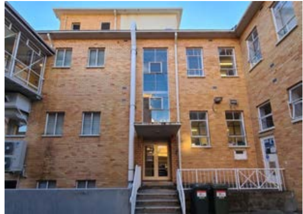
Building 8 – Engineering Building Minor Southern Entrance Source: Paul Davies Pty Ltd
