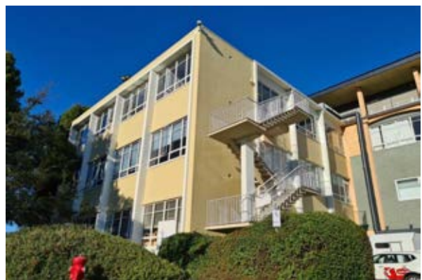
Building 12 – Geography, Geology and CODES North-eastern wing Source: Paul Davies Pty Ltd
