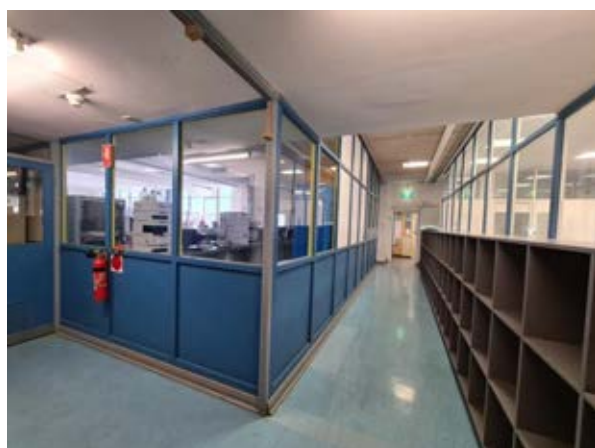
Building 17 - Chemistry, Central Science Laboratory Typical timber joinery to labs
