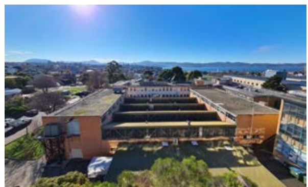
Building 11 – Engineering Workshop View showing the central saw tooth roof form from the roof of the Chemistry Building looking north-east Source: Paul Davies Pty Ltd
