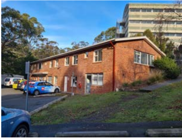
Building 40b – Old Commerce Annex North-eastern corner Source: Paul Davies Pty Ltd
