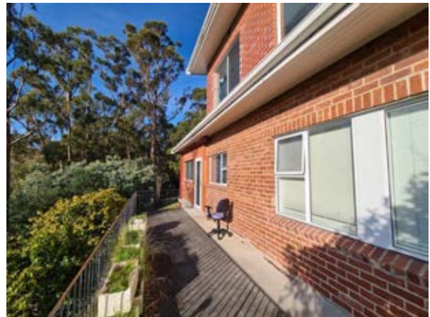
Building 38 – Research House North-eastern façade and open verandah Source: Paul Davies Pty Ltd
