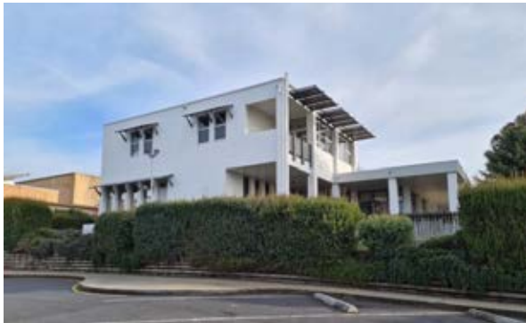
Building 3 – Childcare (Lady Gowrie) North-eastern corner Source: Paul Davies Pty Ltd
