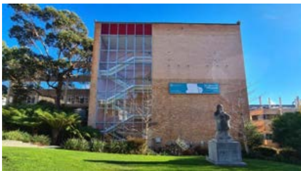
Building 23 – Library, Morris Miller Eastern elevation of the eastern wing, note glazed curtain wall to the stair circulation Source: Paul Davies Pty Ltd
