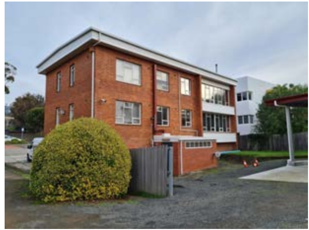
Building 2 – 6 Grace Street North-eastern elevation Source: Paul Davies Pty Ltd
