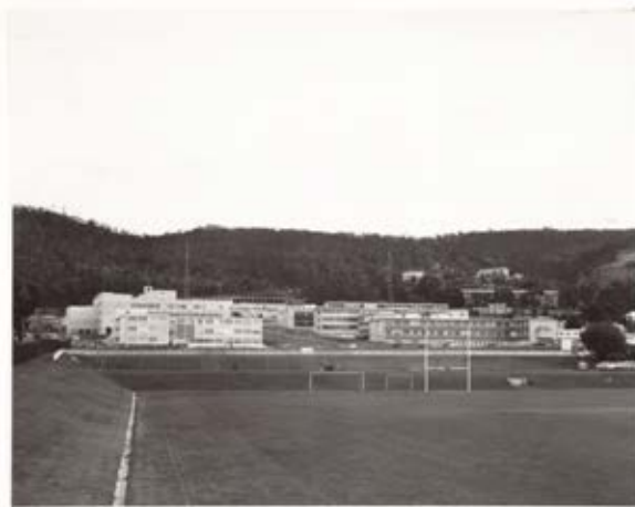
Building 8 – Engineering Building
