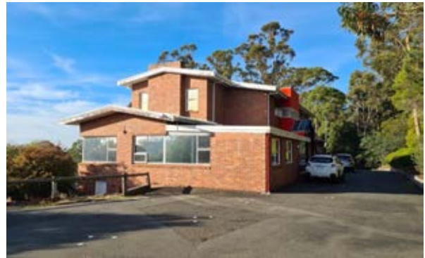
Building 38 – Research House North-western facade Source: Paul Davies Pty Ltd
