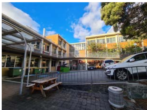
Building 34 – Life Sciences Building Western façade of the 1970-73 southern extension Source: Paul Davies Pty Ltd
