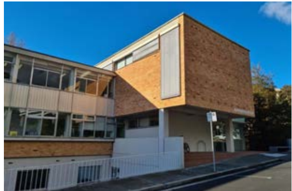
Building 22 – Administration Building First floor cantilever over main entrance Source: Paul Davies Pty Ltd
