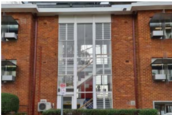
Building 1 – 301 Sandy Bay Road Detail of central stair circulation (South-western elevation) Source: Paul Davies Pty Ltd
