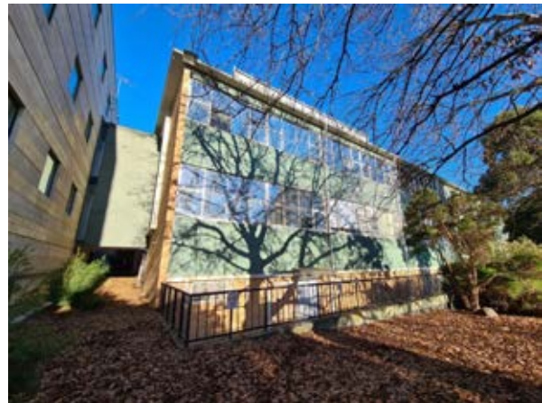
Building 8 – Engineering Building Northern façade (eastern end) Source: Paul Davies Pty Ltd
