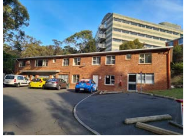
Building 40b – Old Commerce Annex Eastern elevation Source: Paul Davies Pty Ltd
