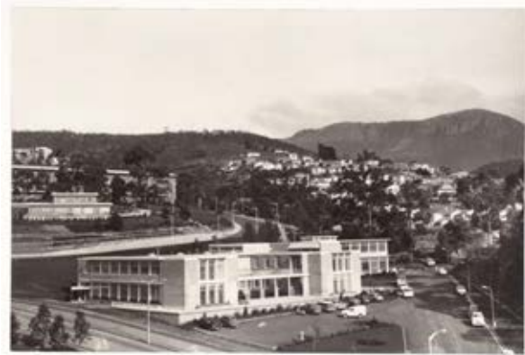
Building 21 – Tasmania University Union (Union Building)
