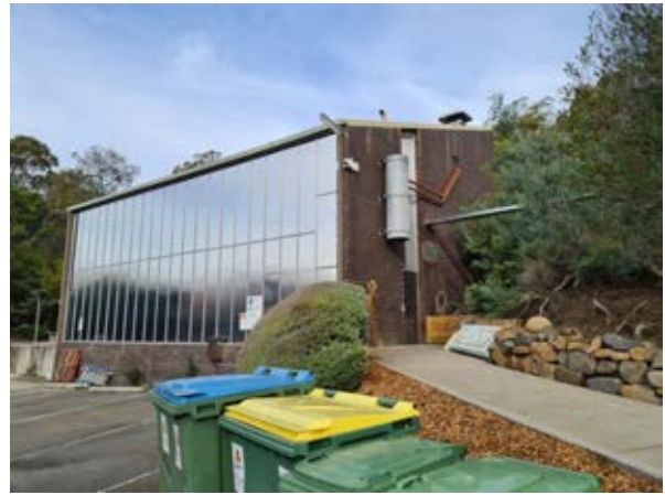
Building 32a – Boiler House Northern elevation Source: Paul Davies Pty Ltd
