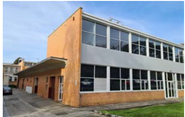
Building 11 – Engineering Workshop North-western corner Source: Paul Davies Pty Ltd
