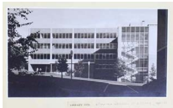
Building 23 – Library, Morris Miller
