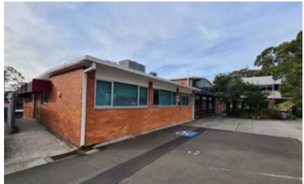
Building 32 – Corporate Services Building South-western corner Source: Paul Davies Pty Ltd
