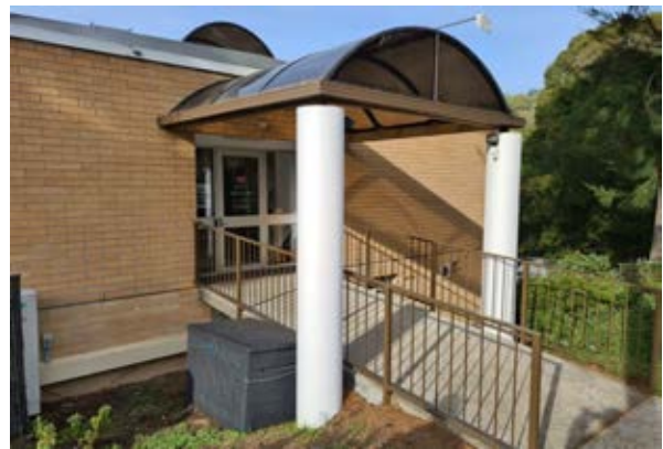
Building 18 – University Club Detail of the rear entrance (Alexander Street) to the 1986 first floor addition. Source: Paul Davies Pty Ltd
