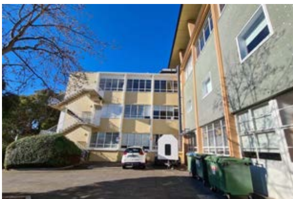
Building 12 – Geography, Geology and CODES North-eastern wing (western façade) Source: Paul Davies Pty Ltd
