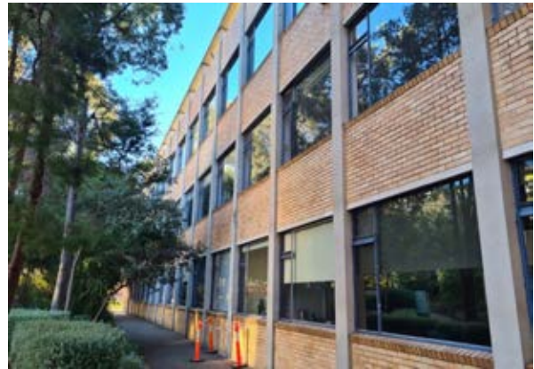
Building 13 – Physics Original North-eastern Façade Source: Paul Davies Pty Ltd
