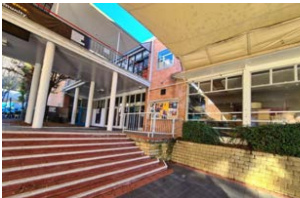
Building 21 – Tasmania University Union View of the two-storey link between the eastern and western wings Source: Paul Davies Pty Ltd
