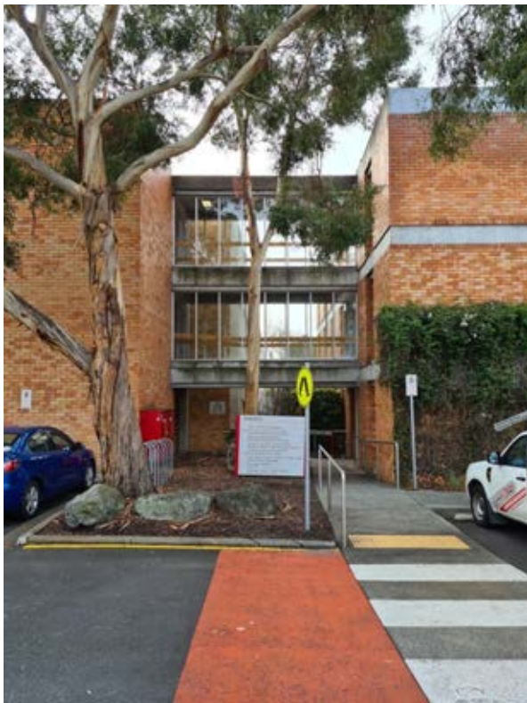
Building 29 – Humanities Building Glazed link between Humanities (image right) and Psychology (image left) - south elevation Source: Paul Davies Pty Ltd
