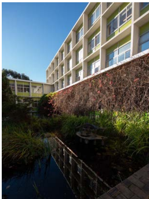
Building 26 – Psychology, Social Sciences Western Façade detail Source: Paul Davies Pty Ltd
