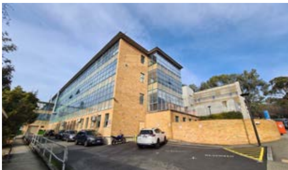
Building 17 - Chemistry, Central Science Laboratory North-western corner Source: Paul Davies Pty Ltd
