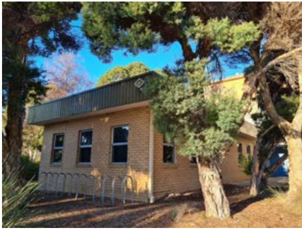
Building 9 – Surveying Building North-western corner, 1989 addition Source: Paul Davies Pty Ltd
