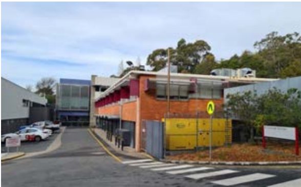
Building 32 – Corporate Services Building Western façade Source: Paul Davies Pty Ltd
