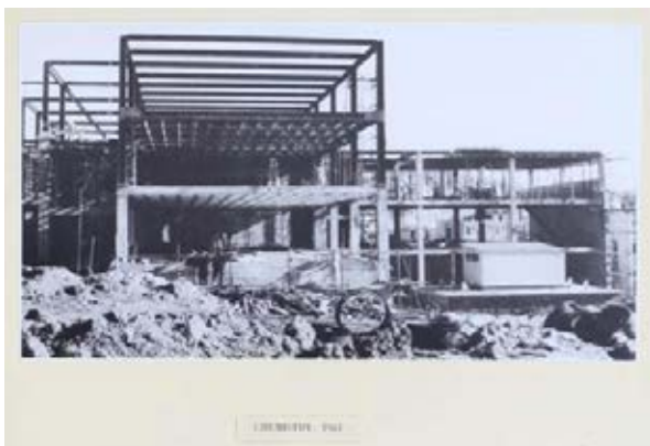
Building 17 - Chemistry, Central Science Laboratory
