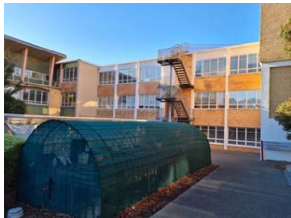
Building 12 – Geography, Geology and CODES Western façade of the eastern wing Source: Paul Davies Pty Ltd
