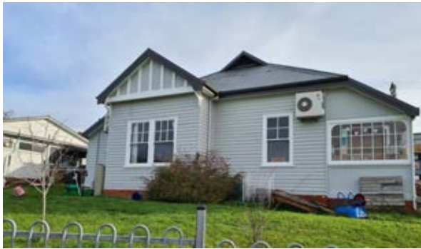
Building 53 – Childcare Cottage South-eastern elevation Source: Paul Davies Pty Ltd
