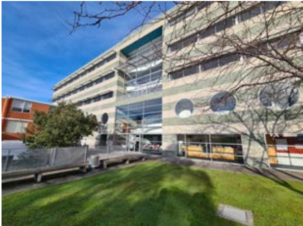
Building 40a – International Pathway College Eastern end of the north-eastern facade Source: Paul Davies Pty Ltd
