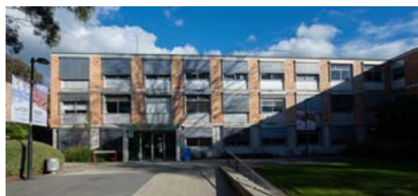
Building 22 – Administration Building Northern elevation, note the original colonnade to ground floor has been infilled. Source: Paul Davies Pty Ltd
