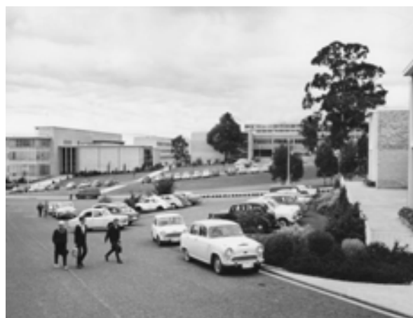
Building 17 - Chemistry, Central Science Laboratory
