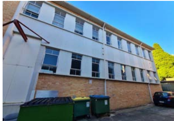
Building 8 – Engineering Building South-eastern wing (eastern façade) Source: Paul Davies Pty Ltd
