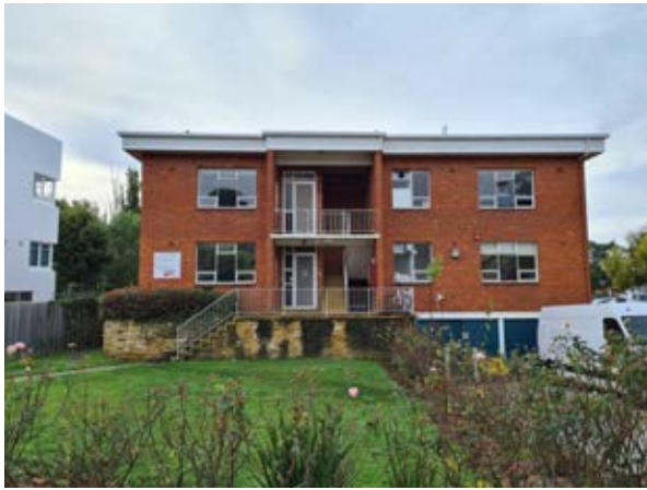
Building 2 – 6 Grace Street South-western elevation (Grace Street Elevation) Source: Paul Davies Pty Ltd
