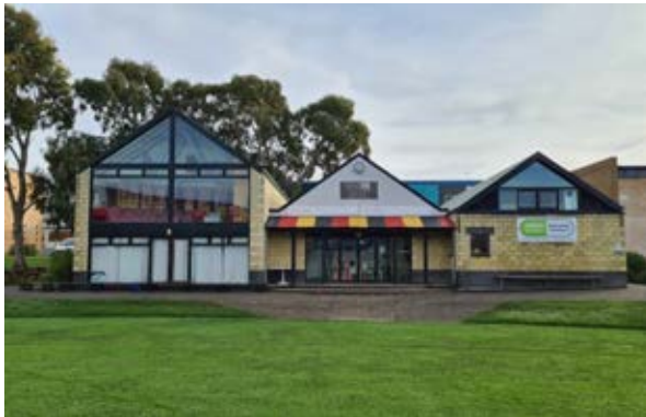
Building 5 – Cricket Pavilion South-eastern elevation (facing oval) Source: Paul Davies Pty Ltd
