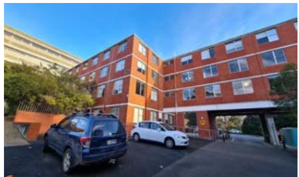
Building 40 – Hytten Hall Eastern façade of the southern extension wing Source: Paul Davies Pty Ltd
