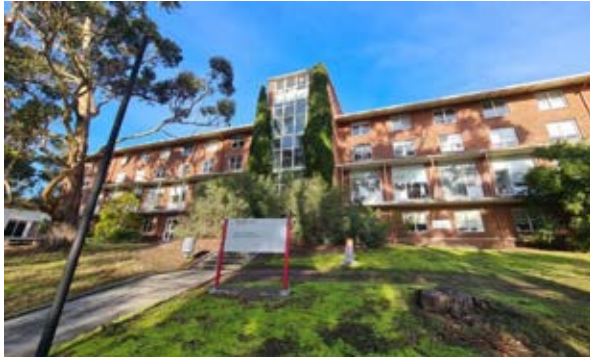
Building 40 – Hytten Hall North-eastern façade Source: Paul Davies Pty Ltd
