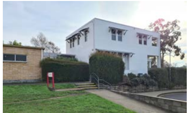
Building 3 – Childcare (Lady Gowrie) South-eastern corner Source: Paul Davies Pty Ltd
