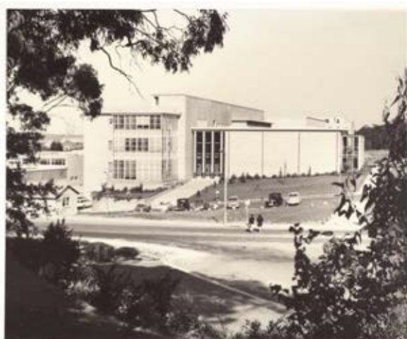
Building 17 - Chemistry, Central Science Laboratory
