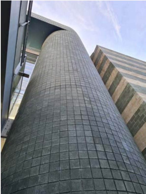
Building 40a –International Pathway College Detail of the large circular columns located on the southern side of the building Source: Paul Davies Pty Ltd
