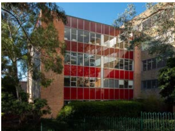
Building 23 – Library, Morris Miller Southern façade of the western wing Source: Paul Davies Pty Ltd
