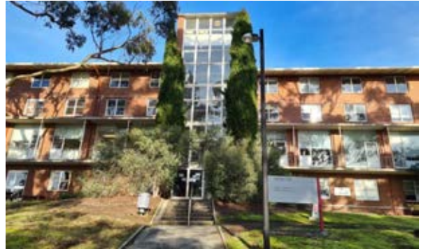
Building 40 – Hytten Hall North-eastern façade, with central glazed staircase and main entrance foyer Source: Paul Davies Pty Ltd
