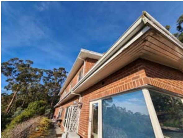
Building 38 – Research House North-eastern facade Source: Paul Davies Pty Ltd
