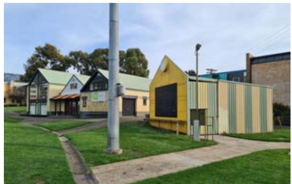
Building 5 – Cricket Pavilion Detail of Cricket Score Board Source: Paul Davies Pty Ltd
