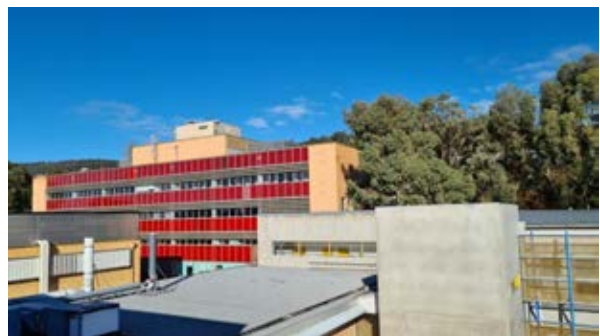
Building 23 – Library, Morris Miller View of the northern elevation of the Library from the Chemistry building rooftop Source: Paul Davies Pty Ltd
