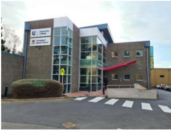
Building 49 – Old IMAS Building
