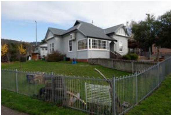
Building 53 – Childcare Cottage South-eastern elevation Source: Paul Davies Pty Ltd
