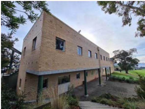
Building 6 – Law Building South-eastern corner, showing the 1988 and 1990 extension. Source: Paul Davies Pty Ltd
