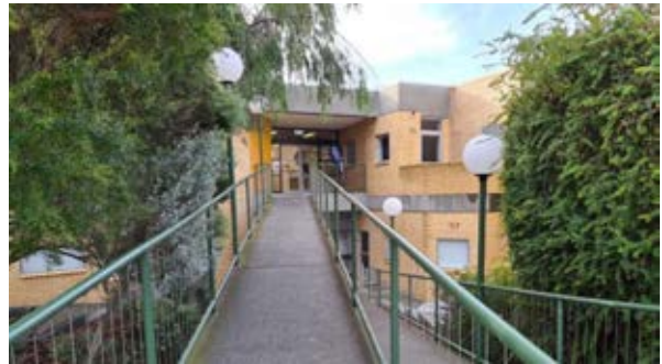
Building 6 – Law Building South-western elevation (main entrance). The concrete entrance ramp was added in 1990. Source: Paul Davies Pty Ltd
