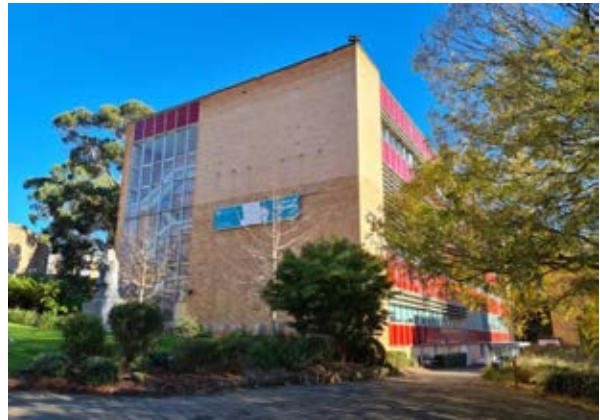
Building 23 – Library, Morris Miller North-eastern corner Source: Paul Davies Pty Ltd
