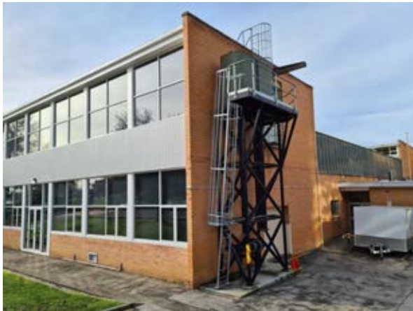
Building 11 – Engineering Workshop South-western corner Source: Paul Davies Pty Ltd
