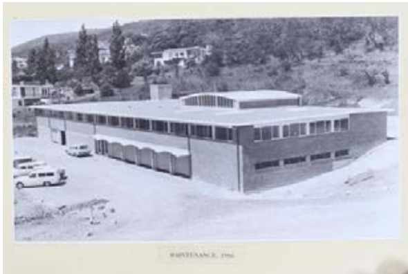
Building 32 – Corporate Services Building (Maintenance Building)
