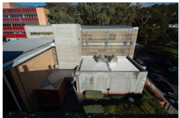
Building 20 - Pharmacy View of the Pharmacy Building from the Chemistry Building rooftop Source: Paul Davies Pty Ltd
