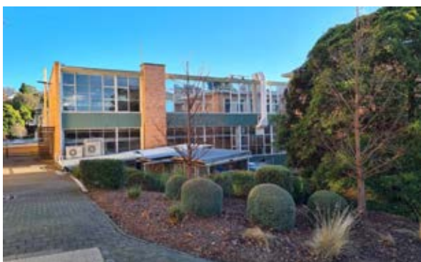
Building 11 – Engineering Workshop Eastern facade Source: Paul Davies Pty Ltd
