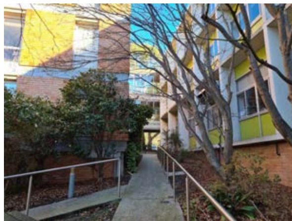
Building 26 – Psychology, Social Sciences Detail of the southern link between the Psychology and Humanities buildings Source: Paul Davies Pty Ltd
