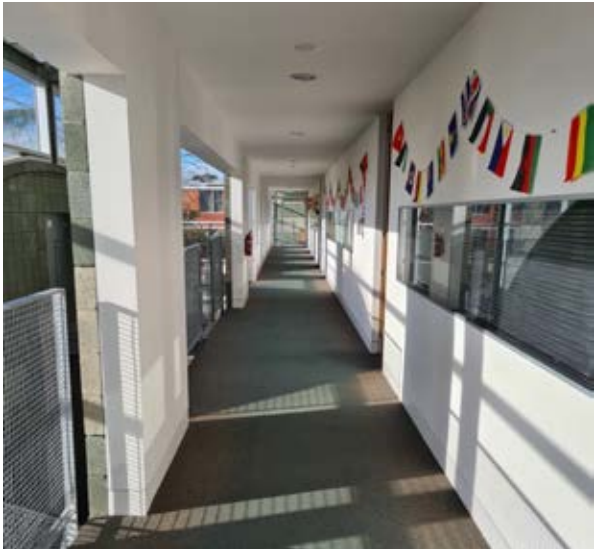
Building 40a –International Pathway College Typical corridor running along the north-eastern side of the building Source: Paul Davies Pty Ltd
