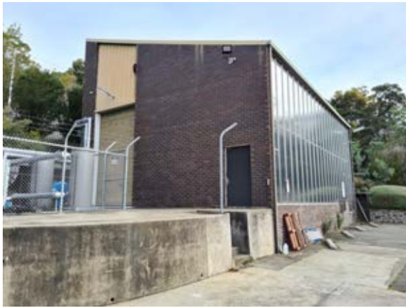
Building 32a – Boiler House Eastern elevation Source: Paul Davies Pty Ltd
