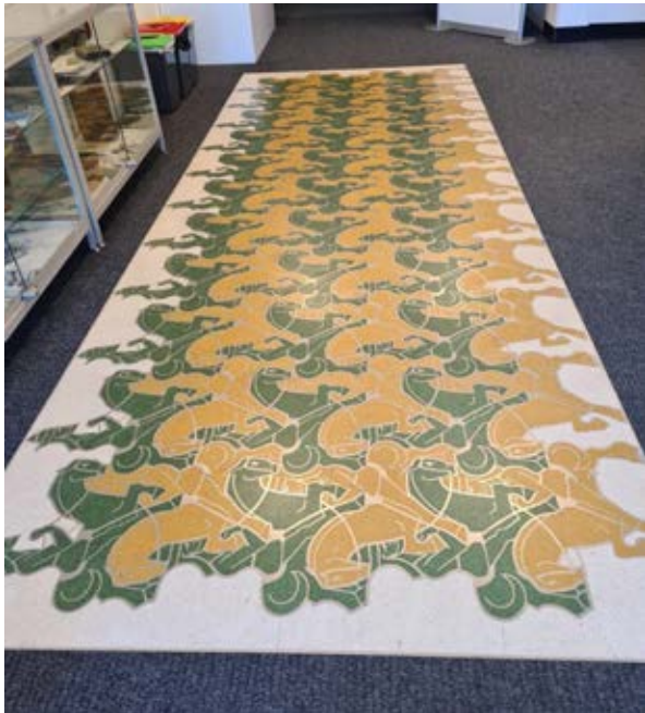
Building 12 – Geography, Geology and CODES Clark Road Entrance Foyer – detailed tessellated terrazzo floor inlay Source: Paul Davies Pty Ltd
