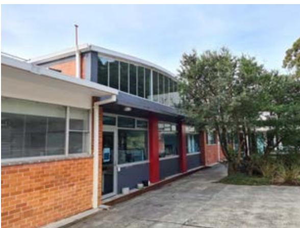
Building 32 – Corporate Services Building Southern façade Source: Paul Davies Pty Ltd
