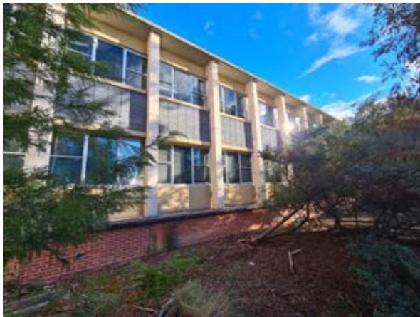
Building 34 – Life Sciences Building Original building – north elevation Source: Paul Davies Pty Ltd
