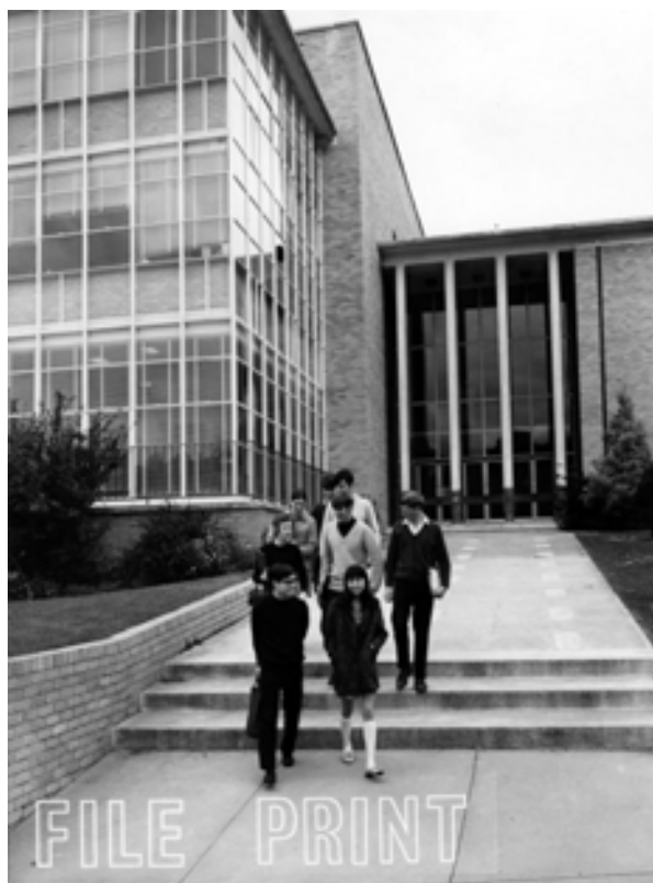
Building 17 - Chemistry, Central Science Laboratory
