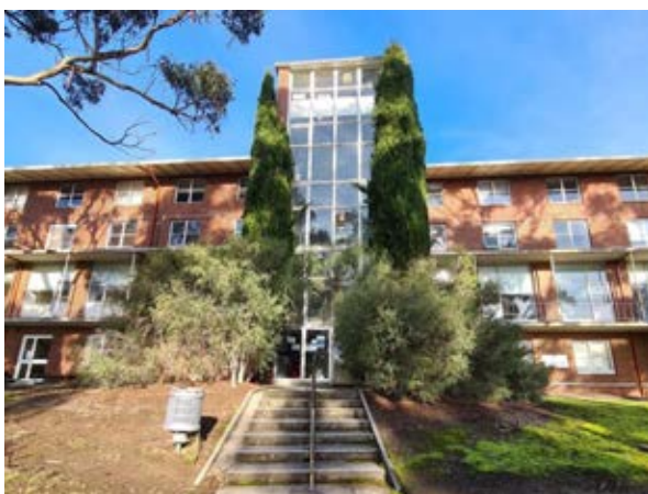
Building 40 – Hytten Hall Central glazed main entrance foyer and staircase Source: Paul Davies Pty Ltd
