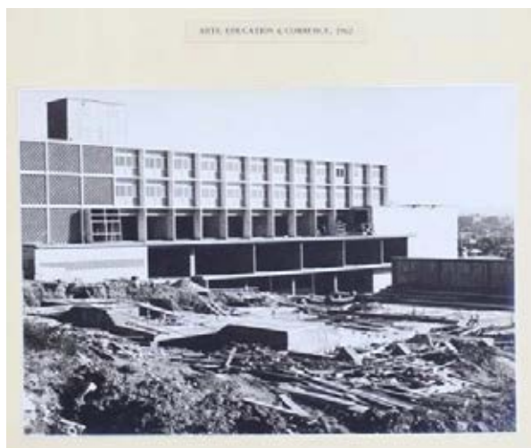
Building 26 – Psychology, Social Sciences (Arts Building) 1962 black and white print Eastern façade, concrete slabs for the Arts Theatre are shown in the foreground Source: University of Tasmania, Collection UT460 – Pictorial History of Sandy Bay Campus Buildings; Item 22
