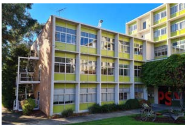
Building 26 – Psychology, Social Sciences Southern façade of the northern wing Source: Paul Davies Pty Ltd
