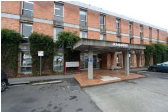
Building 29 – Humanities Building Southern facade Source: Paul Davies Pty Ltd
