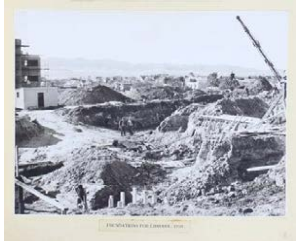
Building 23 – Library, Morris Miller
