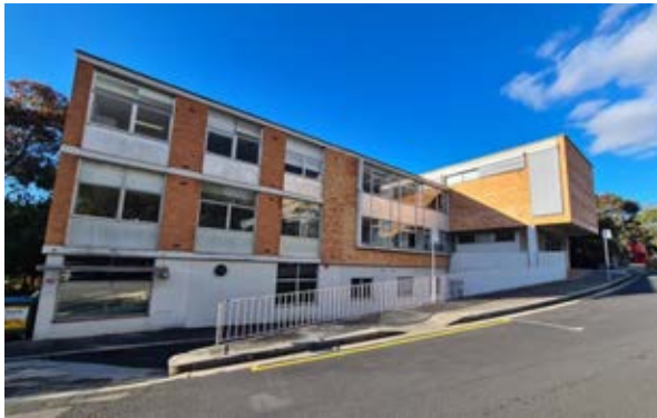
Building 22 – Administration Building Southern Façade facing Dobson Road Source: Paul Davies Pty Ltd
