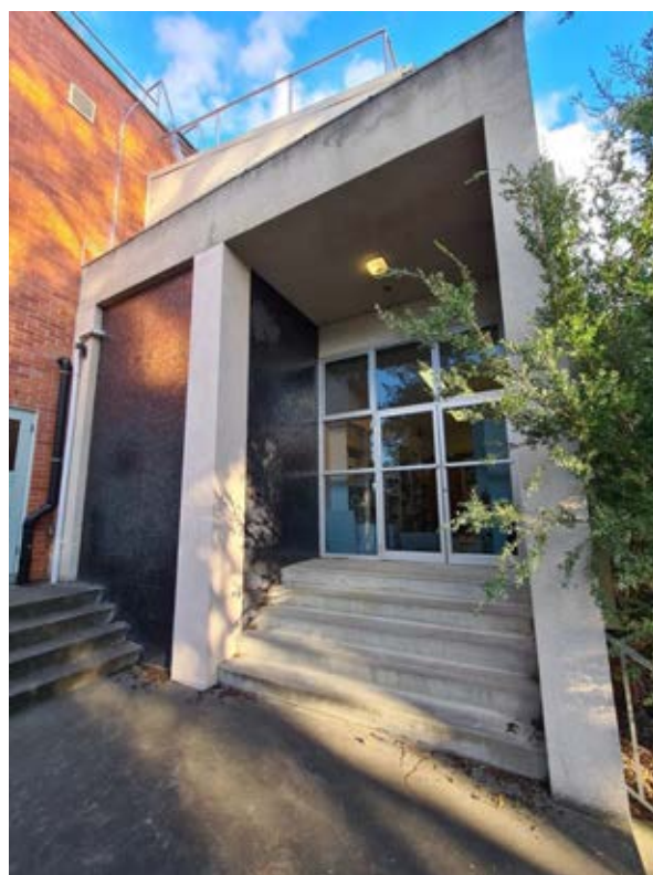
Building 34 – Life Sciences Building Northern façade to the western wing Source: Paul Davies Pty Ltd
