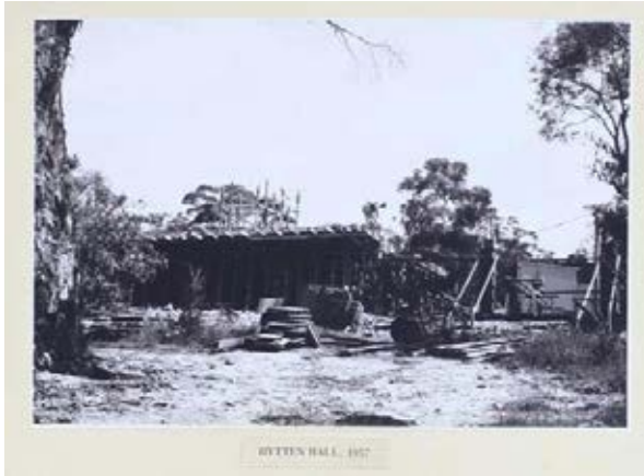
Building 40 – Hytten Hall 1957 black and white print Under Construction
