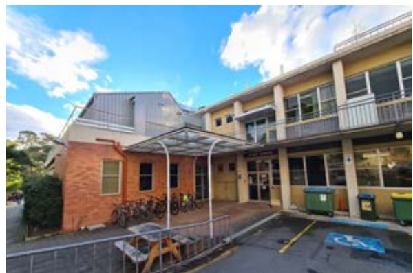
Building 34 – Life Sciences Building South-western corner Source: Paul Davies Pty Ltd
