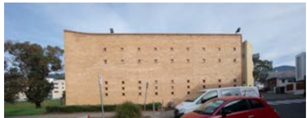
Building 6 – Law Building Northern elevation of the 1989 library extension Source: Paul Davies Pty Ltd
