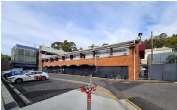
Building 32 – Corporate Services Building Northern façade Source: Paul Davies Pty Ltd
