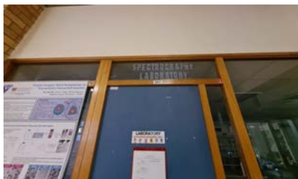
Building 17 - Chemistry, Central Science Laboratory Typical original etched glass signage to the glazed hi-light windows above internal doors.
