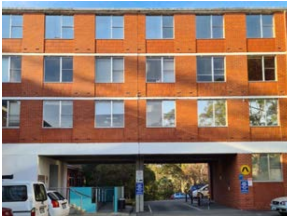
Building 40 – Hytten Hall Detail of the western façade of the southern extension wing. The extension is evident in the brickwork and the double column. Source: Paul Davies Pty Ltd
