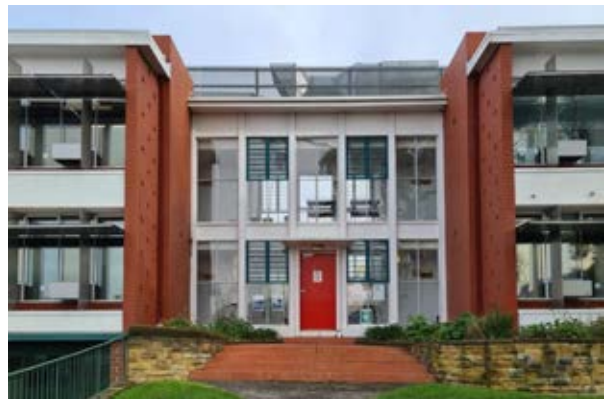
Building 1 – 301 Sandy Bay Road Detail of central stair circulation (Sandy Bay Road elevation) Source: Paul Davies Pty Ltd
