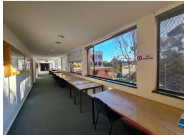
Building 13 – Physics View of a typical internal corridor located on the north-eastern side of the building. Source: Paul Davies Pty Ltd
