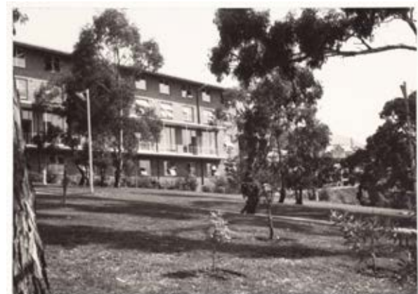
Building 40 – Hytten Hall 1960 Photograph Northern facade
