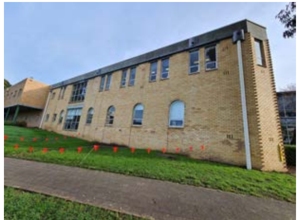
Building 6 – Law Building South-eastern façade. This is the original façade from 1971 however several of the openings were enlarged as part of the 1988 alterations. Source: Paul Davies Pty Ltd
