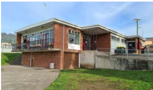
Building 50 – Rugby Pavilion North-eastern corner Source: Paul Davies Pty Ltd
