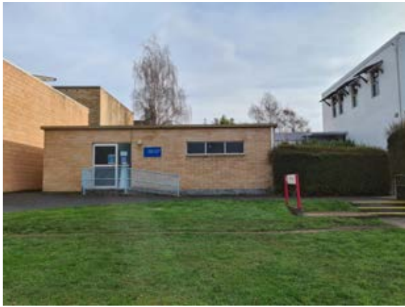
Building 52 – Community Health Clinic
