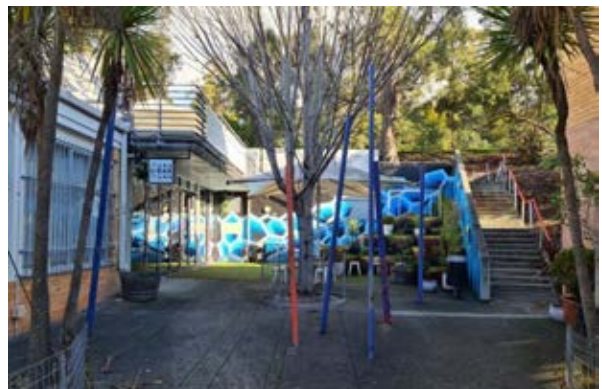
Building 21 – Tasmania University Union View of the south-western courtyard behind the Uni Bar Source: Paul Davies Pty Ltd
