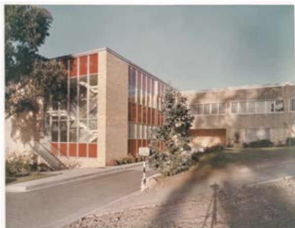
Building 23 – Library, Morris Miller
