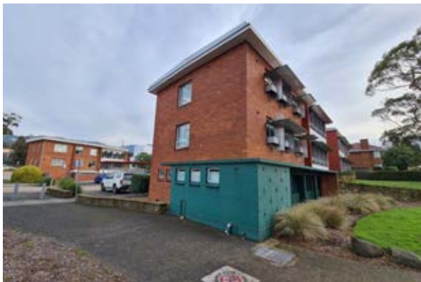
Building 1 – 301 Sandy Bay Road South-eastern elevation Source: Paul Davies Pty Ltd
