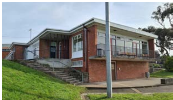
Building 50 – Rugby Pavilion South-eastern corner Source: Paul Davies Pty Ltd
