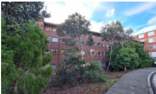
Building 40 – Hytten Hall Southern façade of the original western wing Source: Paul Davies Pty Ltd
