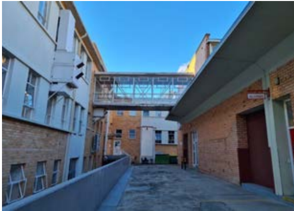
Building 8 – Engineering Building Elevated bridge link between the Engineering Building and the Engineering Workshop Source: Paul Davies Pty Ltd
