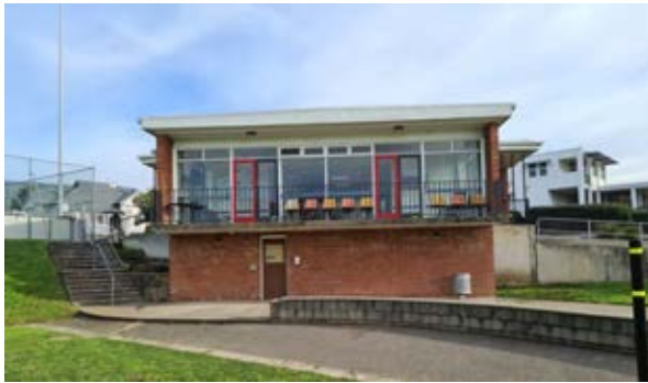
Building 50 – Rugby Pavilion Eastern façade (facing playing field) Source: Paul Davies Pty Ltd
