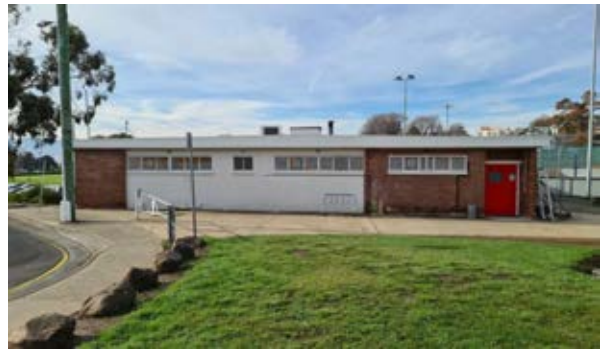
Building 50 – Rugby Pavilion East Elevation Source: Paul Davies Pty Ltd
