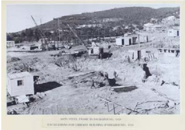
Building 23 – Library, Morris Miller
