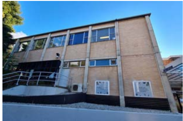
Building 21 – Tasmania University Union Eastern Façade – south-western wing Source: Paul Davies Pty Ltd
