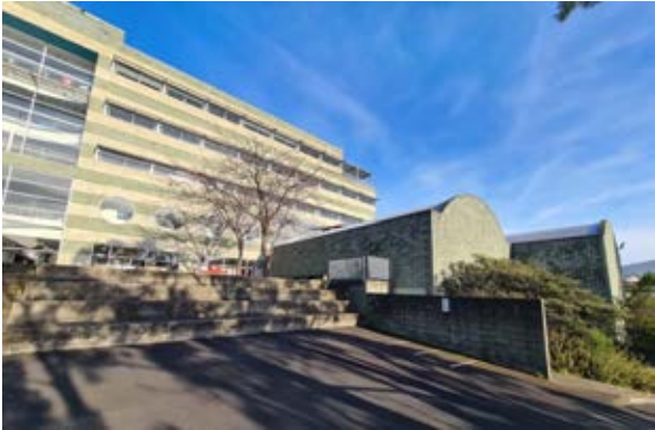
Building 40a – International Pathway College Western end of the north-eastern facade Source: Paul Davies Pty Ltd
