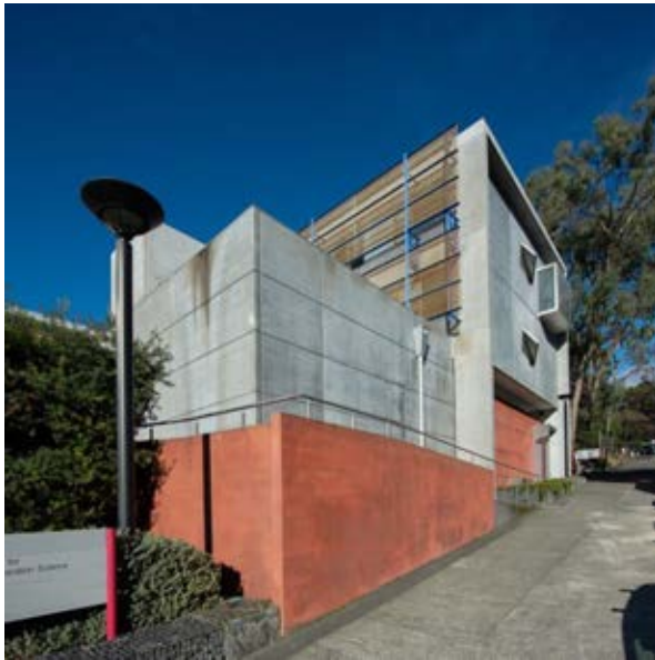
Building 20 - Pharmacy Western façade facing Dobson Road Source: Paul Davies Pty Ltd
