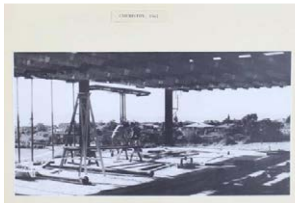
Building 17 - Chemistry, Central Science Laboratory
