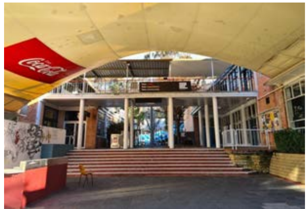
Building 21 – Tasmania University Union Two-storey link between the eastern and western wings and light-weight tensile fabric canopy over the courtyard between the two wings Source: Paul Davies Pty Ltd
