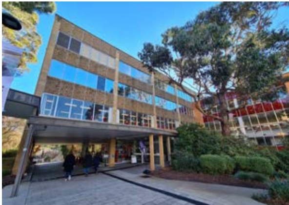
Building 23 – Library, Morris Miller Southern wing and main entrance via building under-croft Source: Paul Davies Pty Ltd
