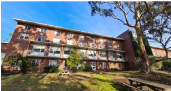
Building 40 – Hytten Hall North-eastern façade of the eastern wing Source: Paul Davies Pty Ltd
