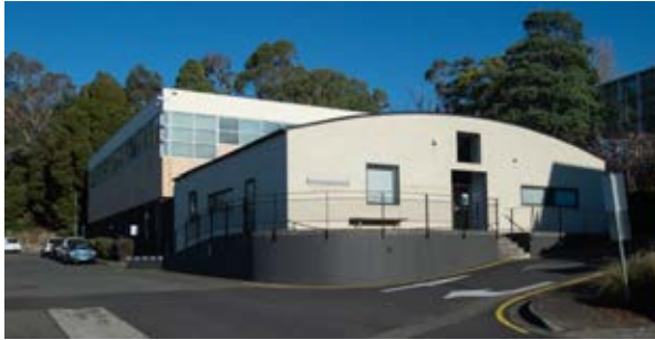
Building 28 – Psychology Research Centre North-eastern corner with the 1990 extension in the foreground Source: Paul Davies Pty Ltd
