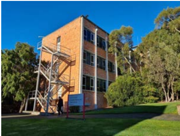
Building 14 – Mathematics Northern-western corner, showing the external steel fire stair. Source: Paul Davies Pty Ltd
