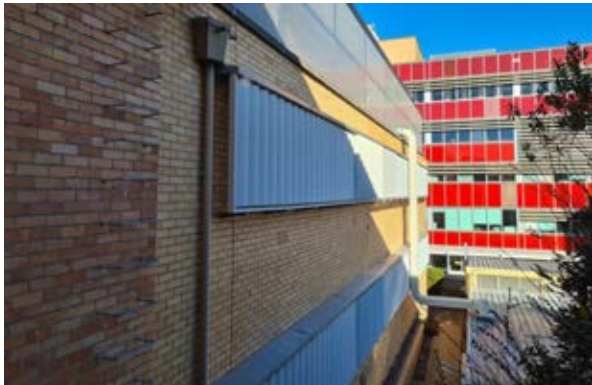
Building 17 - Chemistry, Central Science Laboratory Western façade of the southern wing Source: Paul Davies Pty Ltd
