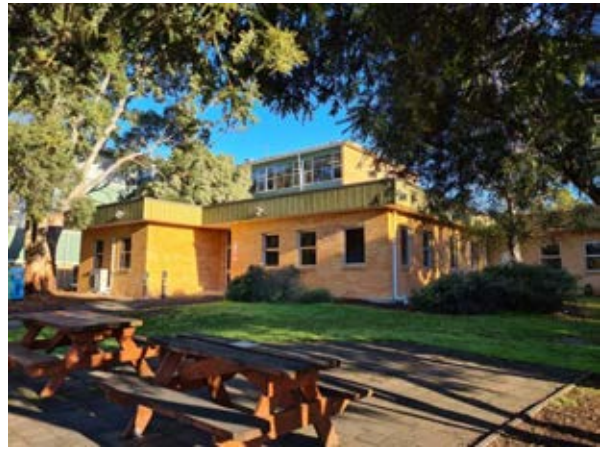
Building 9 – Surveying Building North-eastern corner, original 1979 building Source: Paul Davies Pty Ltd
