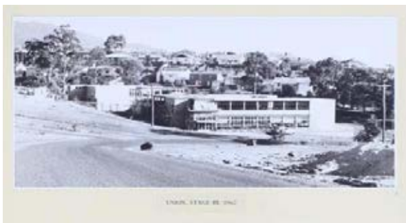
Building 21 – Tasmania University Union (Union Building) Union Building : Stage 3 1962 black and white print Eastern facade Source: University of Tasmania, Collection UT460 – Pictorial History of Sandy Bay Campus Buildings; Item 35
