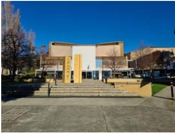
Building 25 – University Centre
