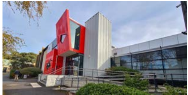
Building 4 – Uni Gym South-eastern facade Source: Paul Davies Pty Ltd
