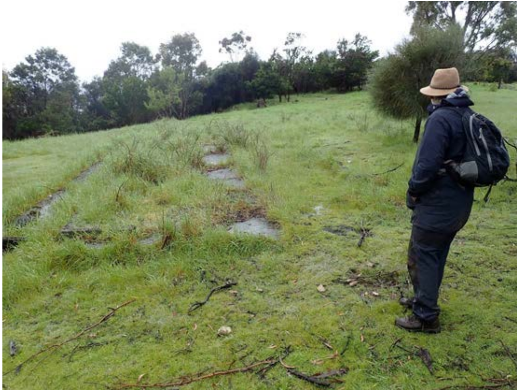
Plate 3: View north across the central property showing typical topography and vegetation structure and one of numerous building foundations
