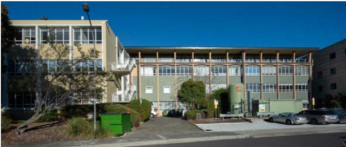
Figure 21: Geology Building with the much later upper floor addition and an early wing to the left of photo. Source: Paul Davies Pty Ltd, 2021
