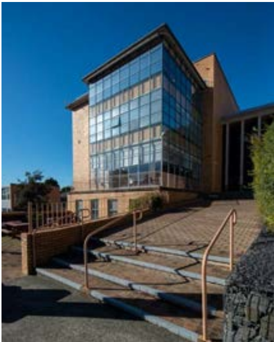
Figure 16: Chemistry Building main entry and glazed curtain wall northern façade.
