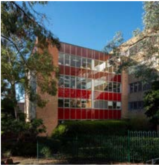
Figure 18: Morris Miller Library curtain wall façade set between brick end walls of the north-south wing.
