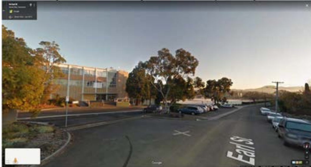
Figure 67 Google Images Capture Jun 2015 Earl Street Sandy Bay looking north east toward Battery Point.
