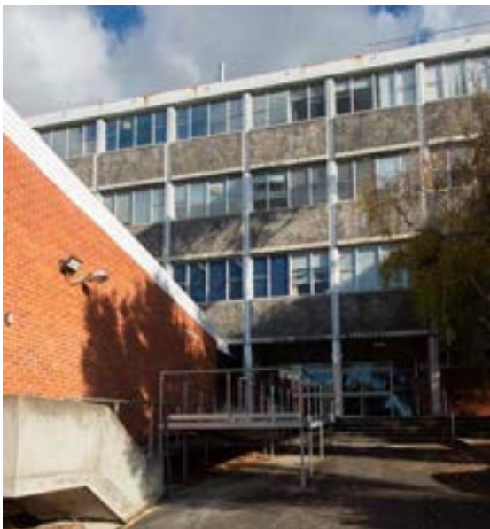
Figure 19: Medical Sciences Building with pre-cast spandrel panels and a later lecture theatre addition to the left.
