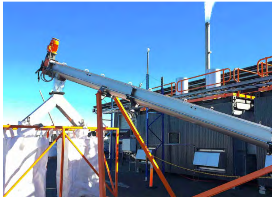
Figure 5: Logan City bio-waste plant (source: ARENA)
